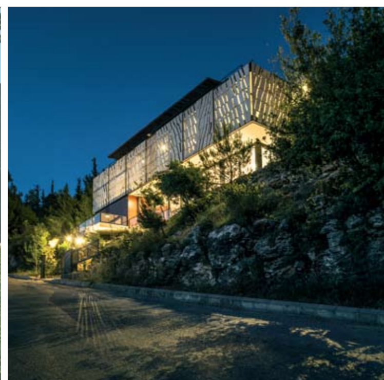
from above to below, from left to right: view from garden towards living area, garden, view from the street at night
